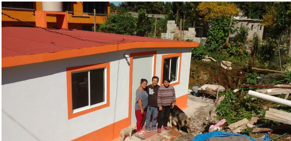
VISTA FACHADA PRINCIPAL
