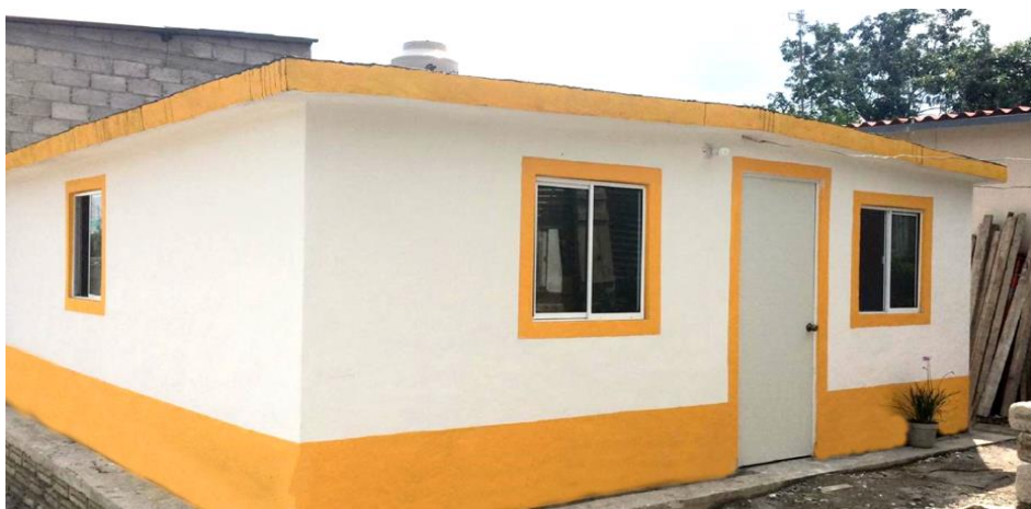
VISTA FACHADA PRINCIPAL
