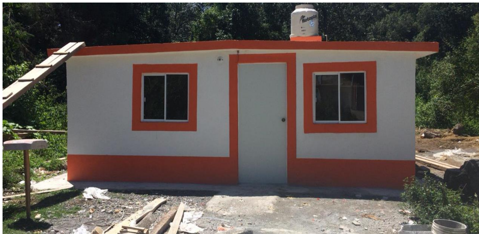
VISTA FACHADA PRINCIPAL
