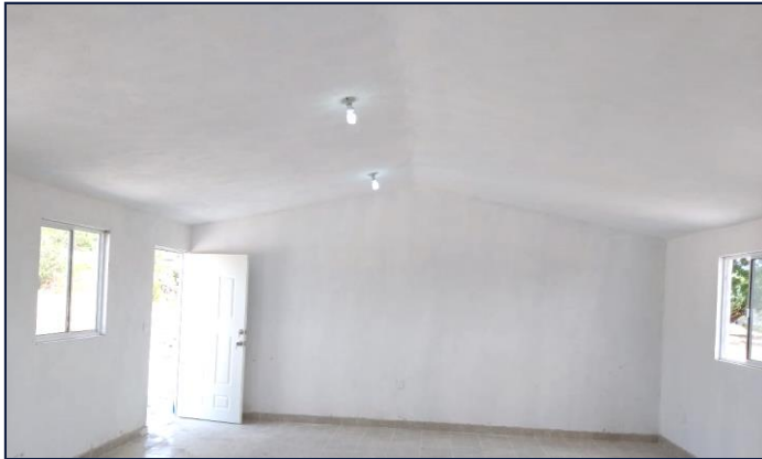
VISTA INTERIOR (AULA 1)
