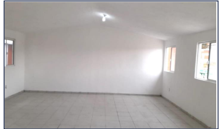
VISTA INTERIOR (AULA 2)
